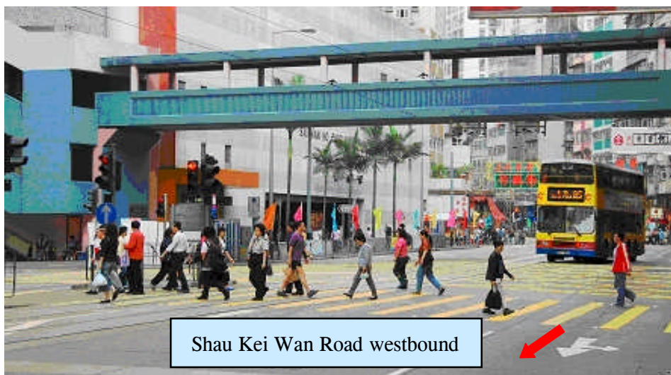
Photograph 6 Footbridge C in Sai Wan Ho
