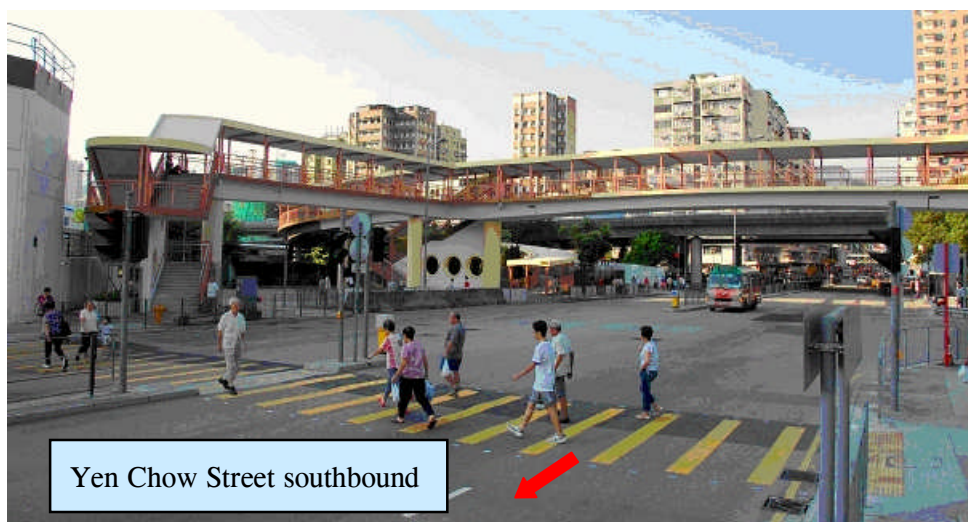
Photograph 3 Footbridge A in Sham Shui Po
