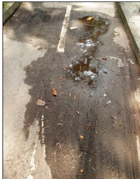
Ting Kok Road near Tai Ping Industrial Estate
