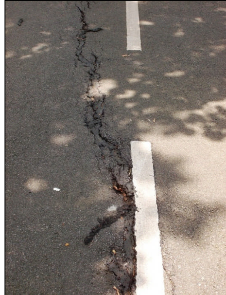
Ting Kok Road near Tai Po Industrial Estate
