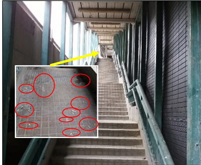
An enclosed staircase with cigarette butts
