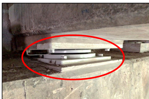
(c) 更換損毀的軸承
