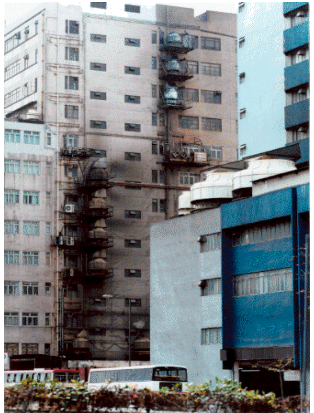
Photograph 6 Large and small cooling towers installed in industrial buildings in Kwun Tong (paragraph 6.28 refers)
