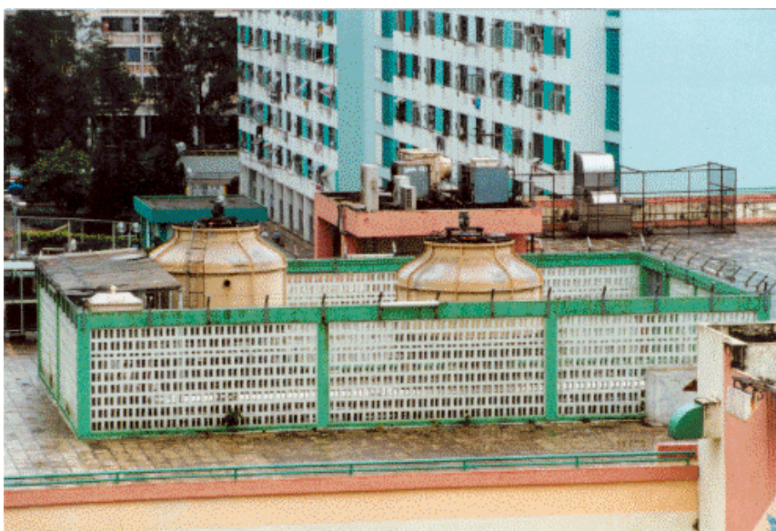
Photograph 4 Two big cooling towers installed on the podium of a public housing estate in Sha Tin (paragraph 6.28 refers)
