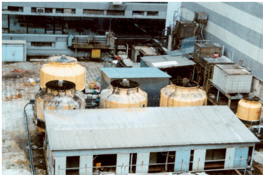
Photograph 3 Old and new cooling towers installed on the podium of a commercial building in Mong Kok (paragraph 6.28 refers)
