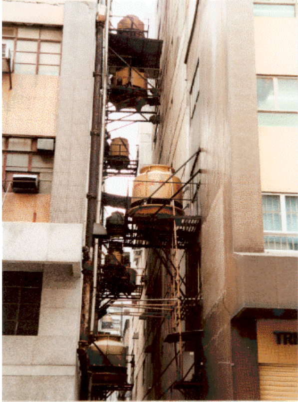
Photograph 6 Large and small cooling towers installed in industrial buildings in Kwun Tong (paragraph 6.28 refers)
