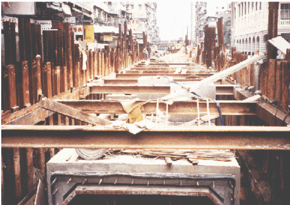
A box culvert under construction in Yen Chow Street
