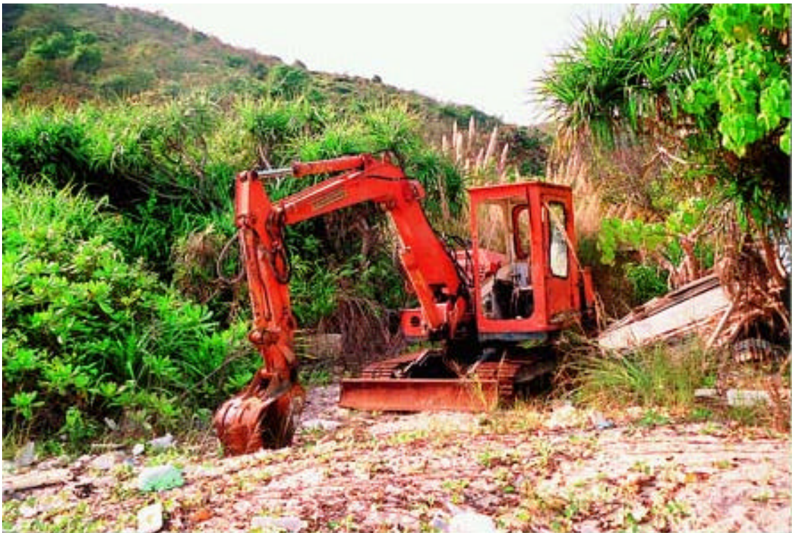
Photograph 4 Excavator and constructional materials found at Ngau Kwu Wan Beach, Lantau Island on 16 January 2002 (para. 5.8 refers)
