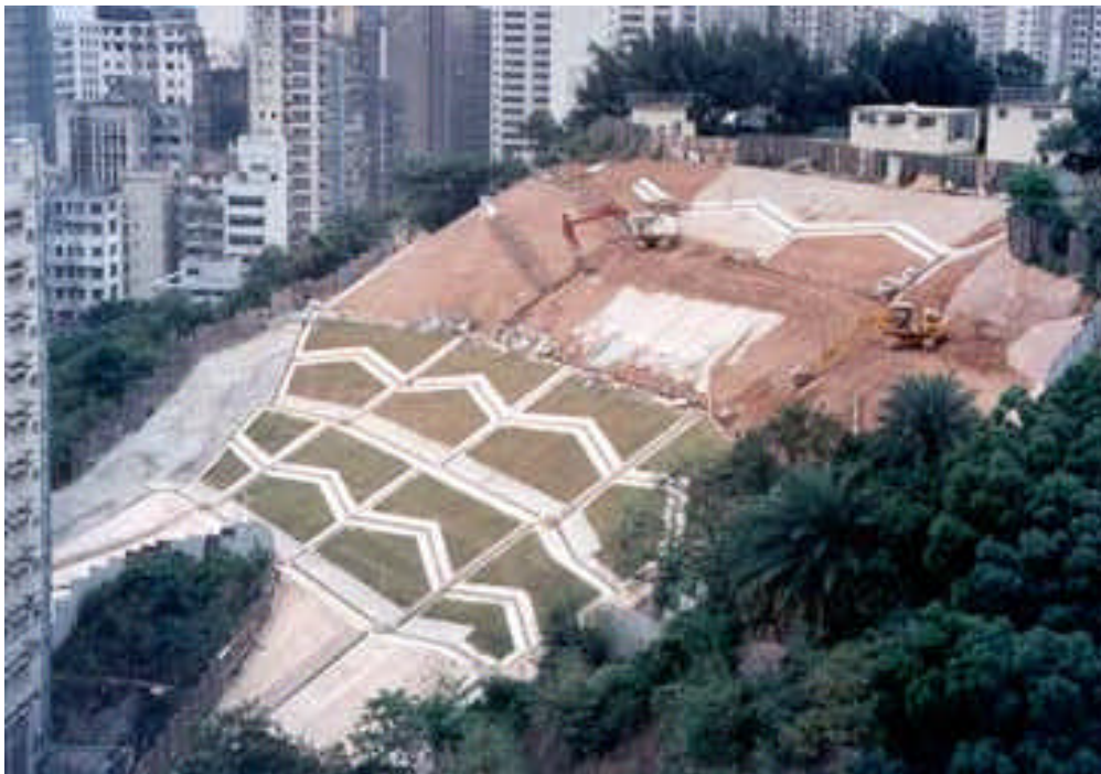
Photograph 2 Slope upgrading works in progress (para. 1.5 refers)
