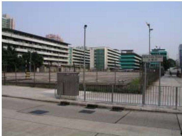
Cheung Sha Wan Factory Estate
