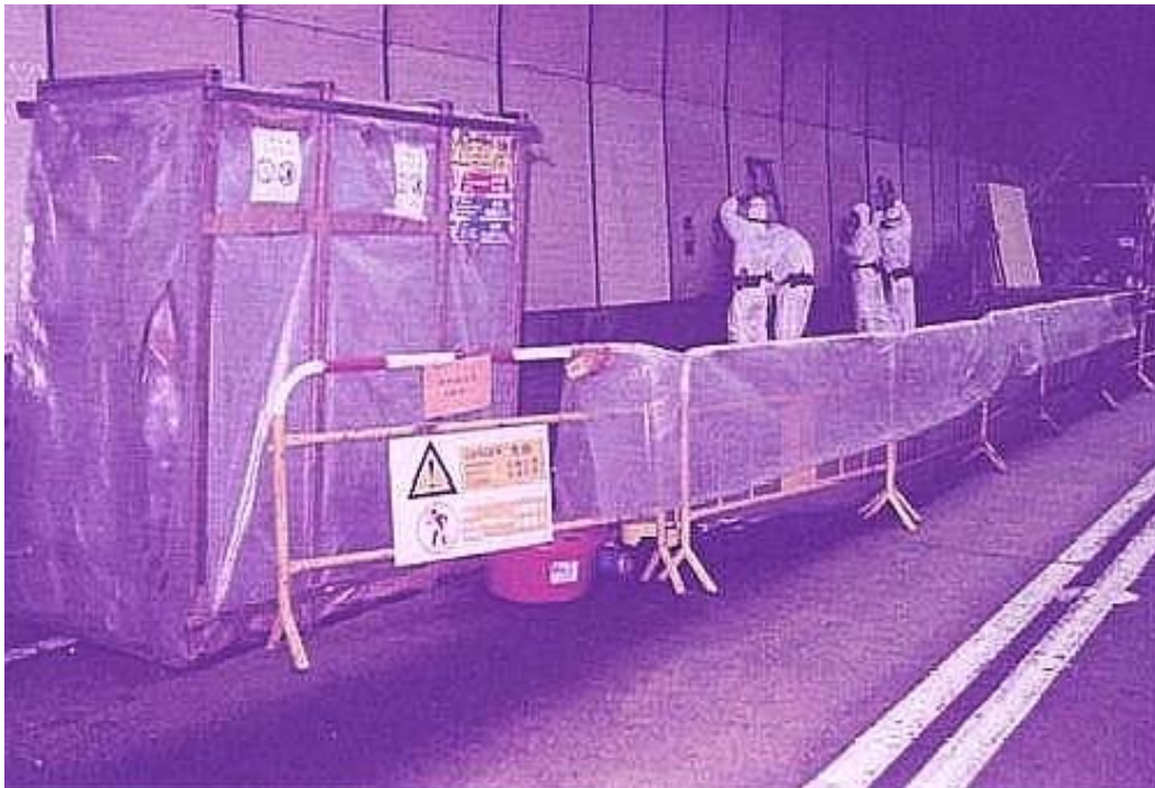
Panel replacement works in the Aberdeen Tunnel
