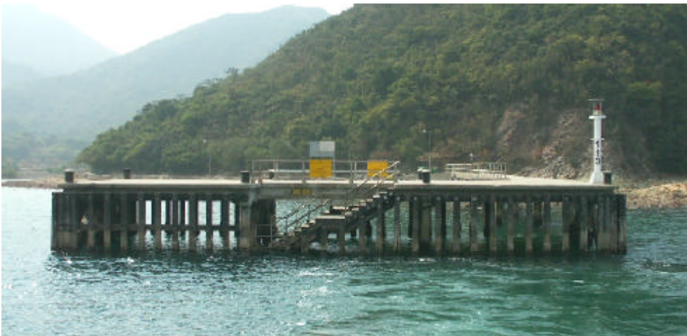
A reinforced concrete pier (Lai Chi Chong Public Pier)
