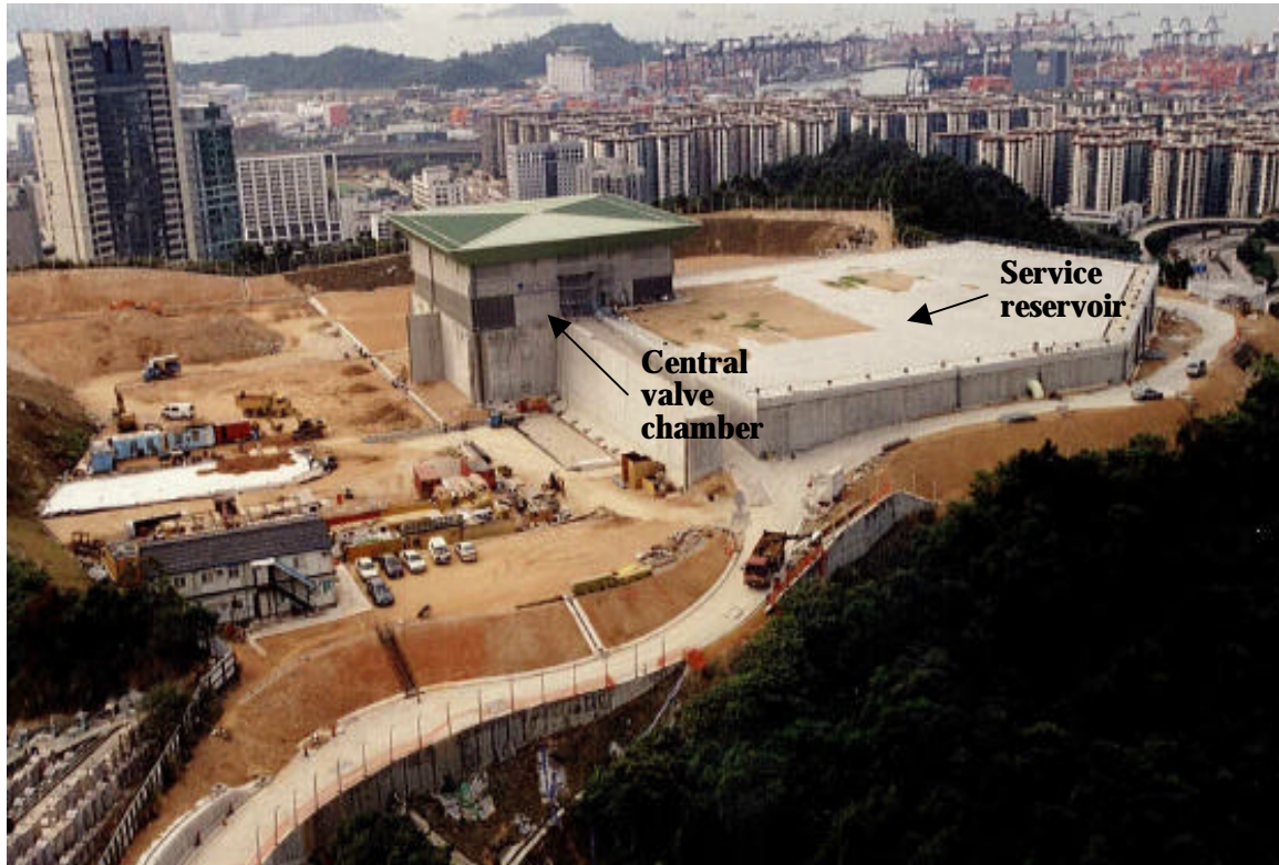
Photograph 1 Butterfly Valley Service Reservoir construction site
