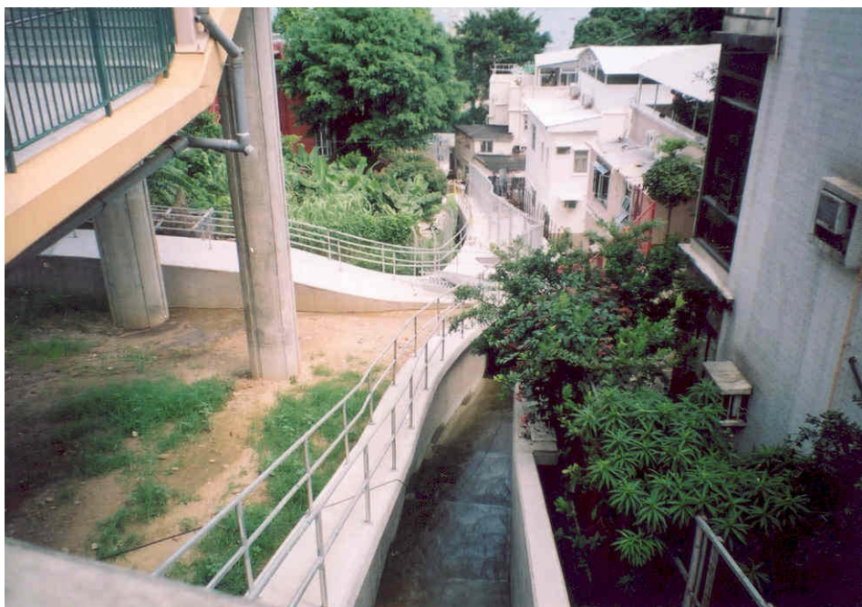
Rainwater channel near Ting Kau Village after improvement works (August 2007)
