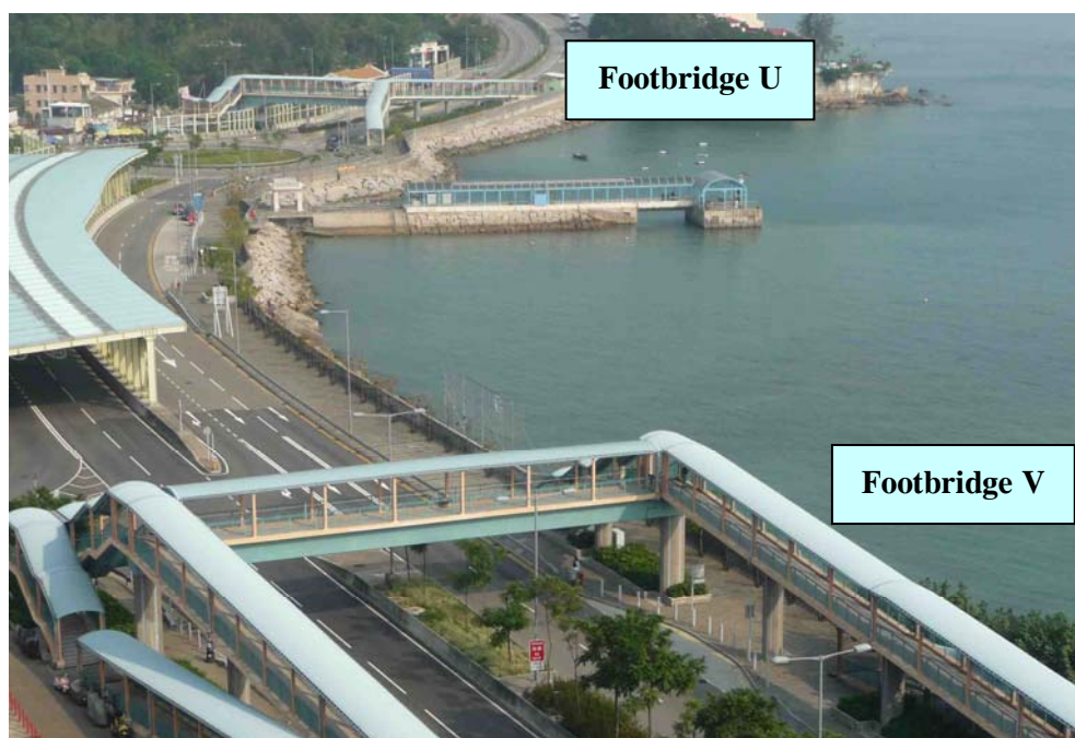
Footbridges U and V in Tsing Lung Tau
