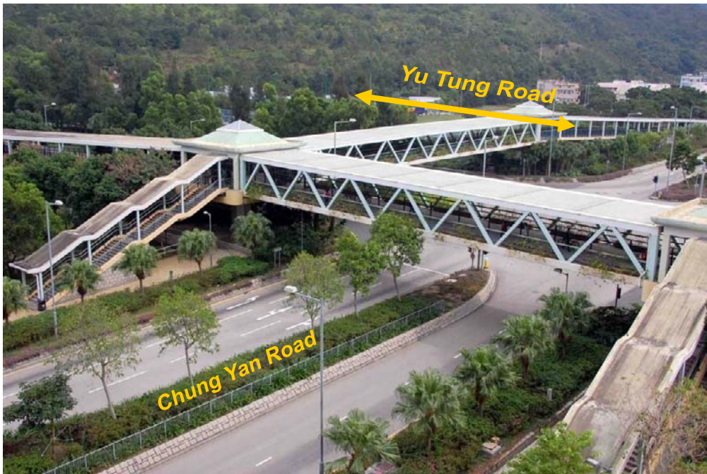
Footbridge K in Tung Chung West
