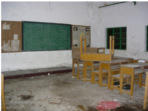
Inside view of the premises
