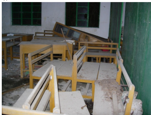
Another inside view of the premises
