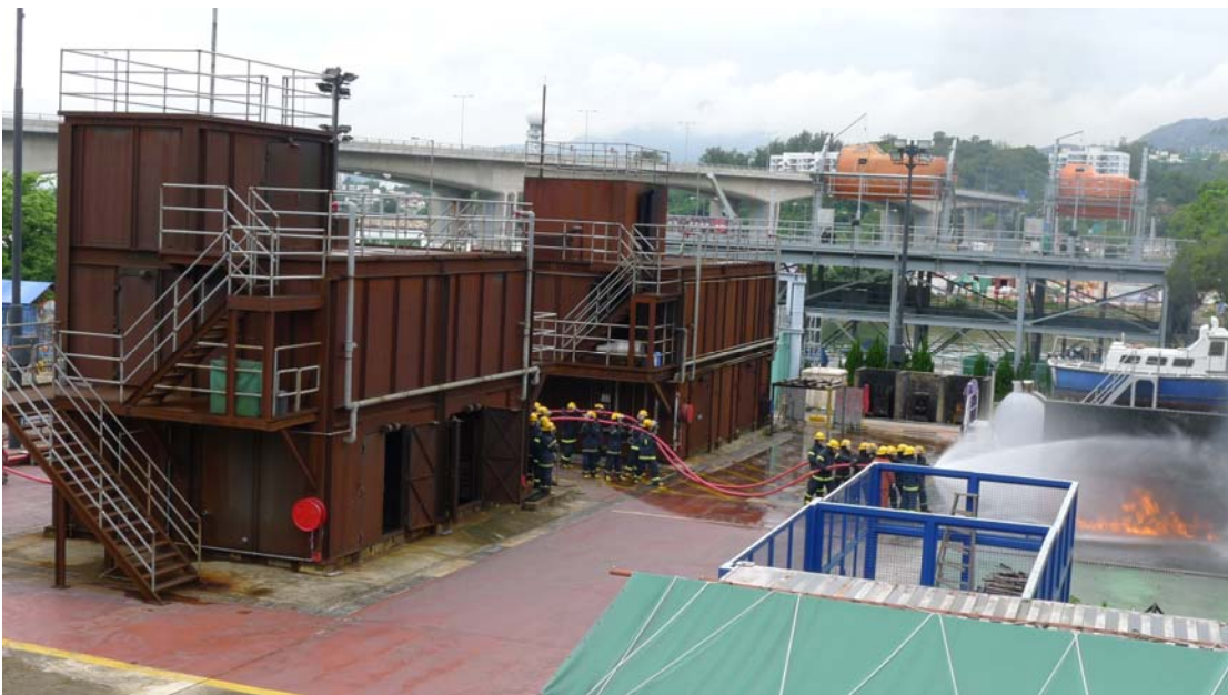
Fire fighting training area
