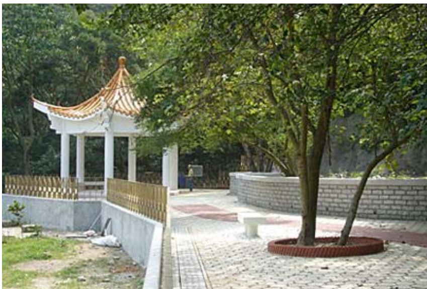
A pavilion constructed under the RPW Programme
