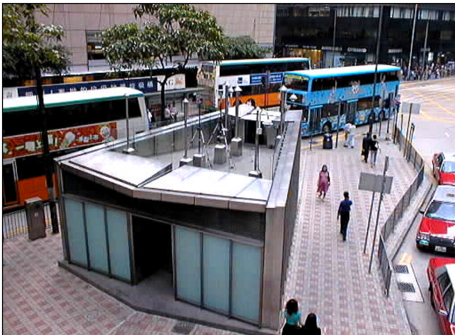
A roadside air-quality monitoring station in Central
