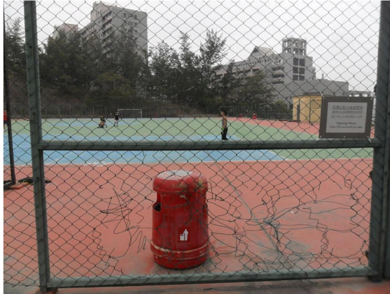
Wire fence which had possibly been vandalised
