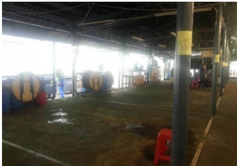
Vacant stalls in Ma Kok Street CFHB
