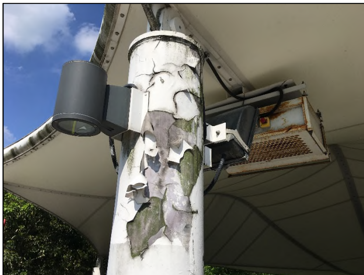
Column with paint peeled off at amphitheatre
