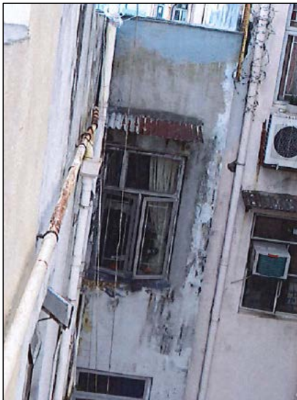
(c) Water pipes with stains at building exterior
