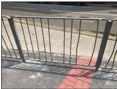
(c) Damaged railings at Hoi Bun Road
