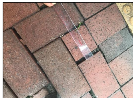
(f) Gap wider than 10 mm between paving blocks at Battery Street
