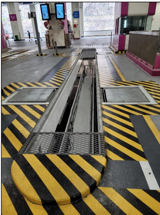
(c) An air-conditioned vehicle examination pit
