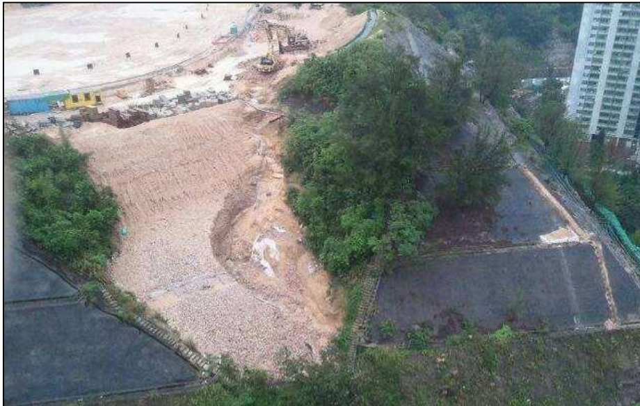
Landslide occurred on a slope (22 May 2013)
