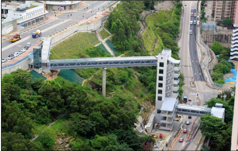
Footbridge B (June 2016)
