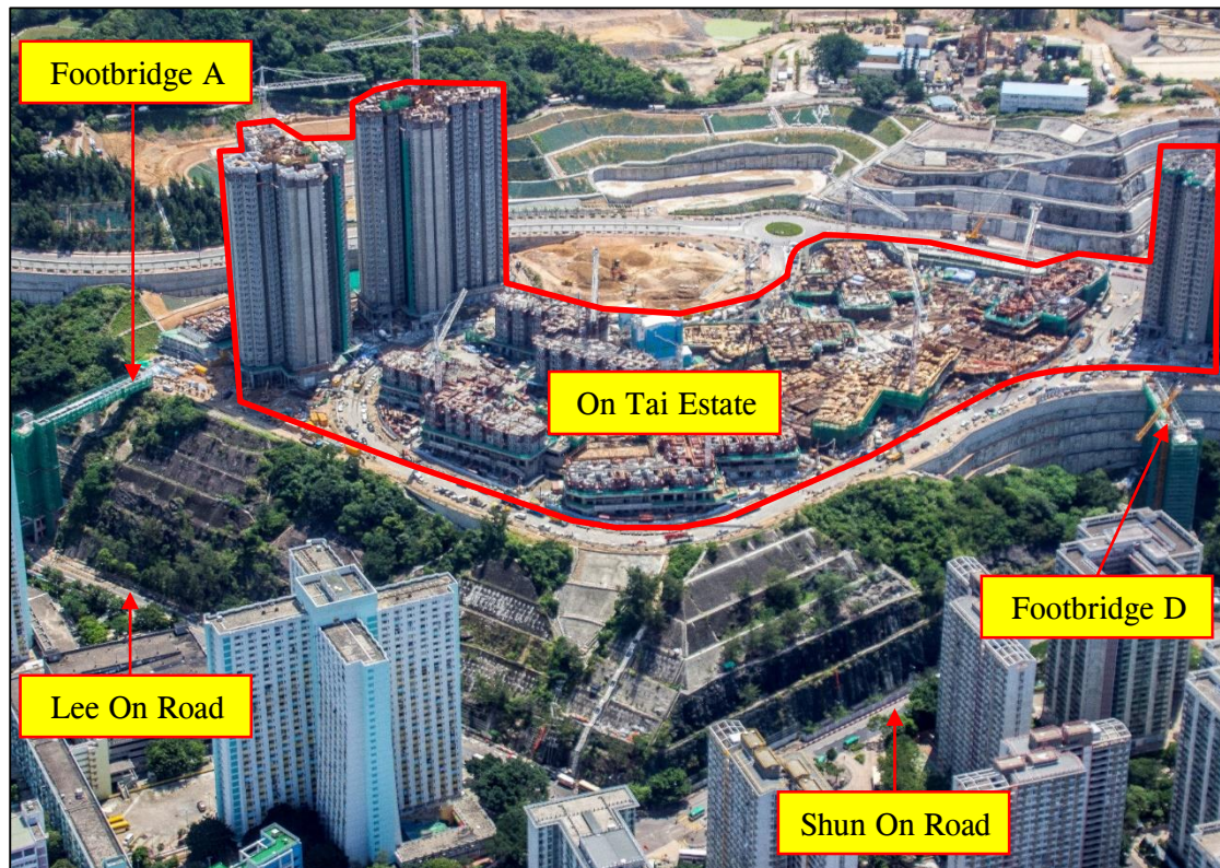
Footbridges A and D (July 2016)
