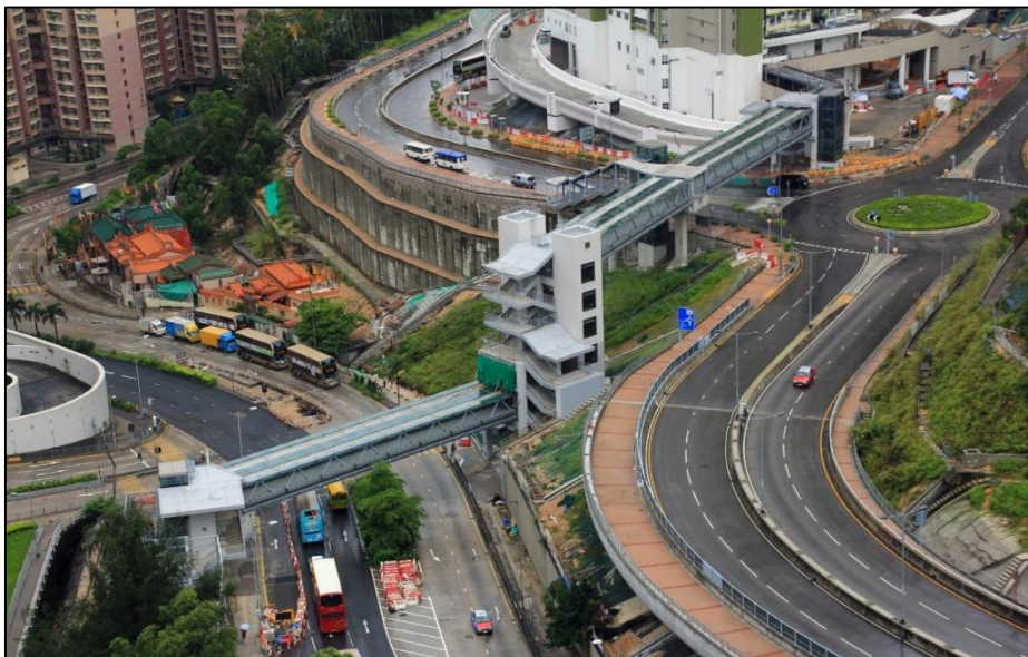
Footbridge C (June 2016)
