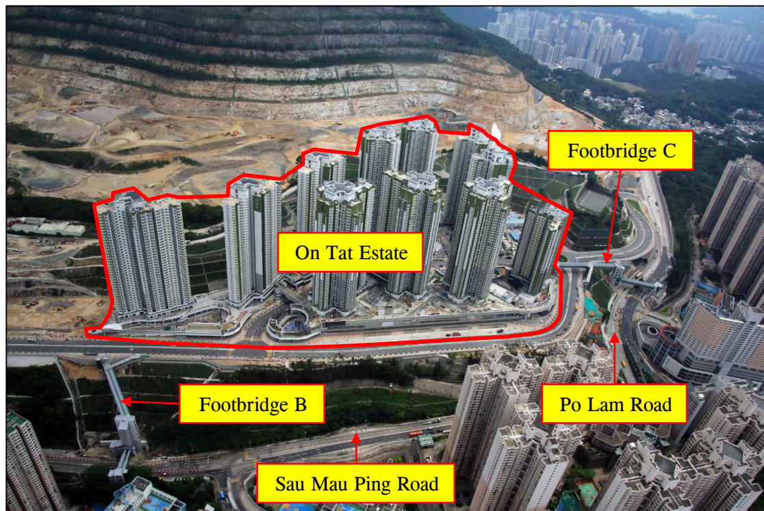
Footbridges B and C (April 2016)
