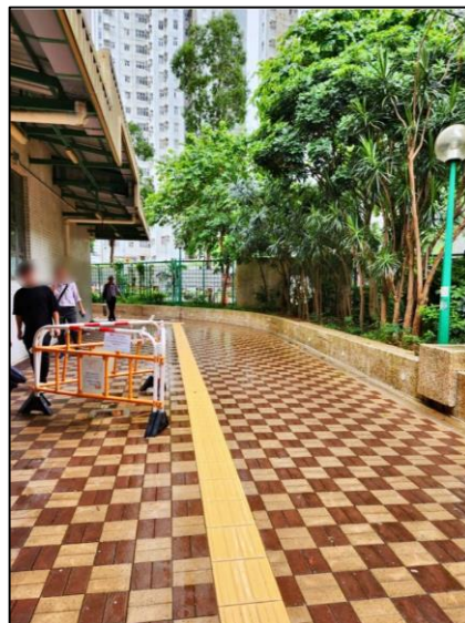
(b) Tactile guide path not under cover
