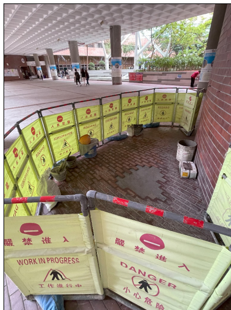
(b) Repair and maintenance work for floor tiles
