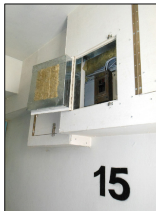
(b) Cable and duct protection
