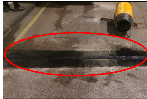
(b) Replacement of defective movement joints
