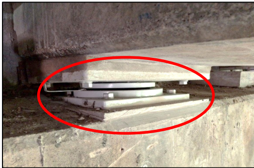
(c) Replacement of a defective bearing
